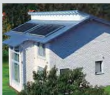
Architect's own home, Bad Füssing, Germany
