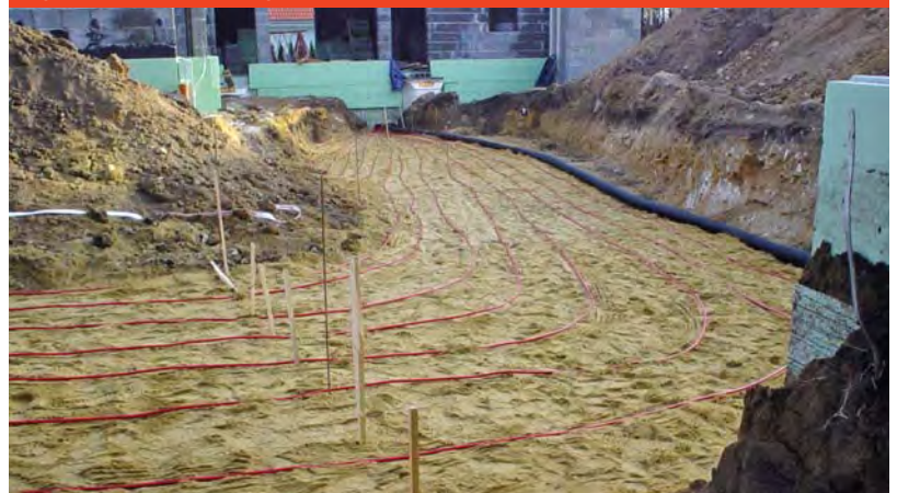
Fig. A.4.1-2 Heat source – geothermal collector
