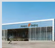
Ameco A380 Hangar Beijing, China
