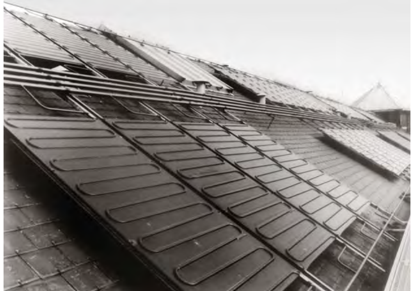
Fig. A.4.6-1 Heat source – non-glazed absorber
