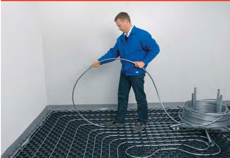
Fig. D.2.2-6 Area heating systems
