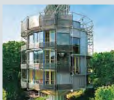
Heliotrop Freiburg, Germany
