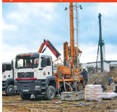
Fig. A.4.1-6 Geothermal probe borehole
