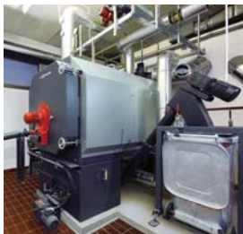
Commercial academy and school, Lustenau, Austria – Vitoflex 300-RF with 220 kW rated heating output
