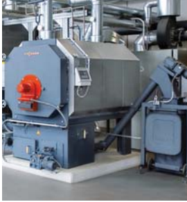
Vitoflex 300-RF wood boiler with rotation combustion for pellets, woodchips and wood shavings
